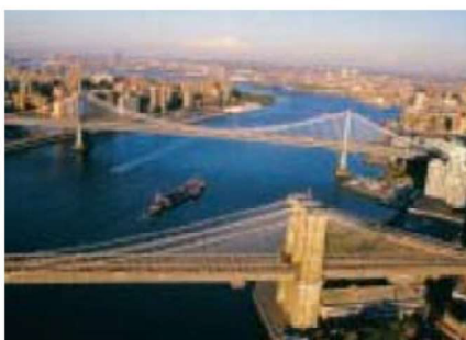
FIGURE 12-30 Suspension bridges (Brooklyn and Manhattan bridges, NY).
