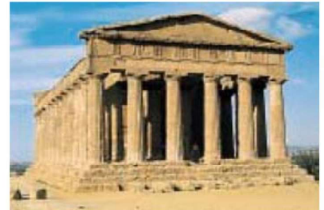
FIGURE 12–17 This Greek temple, in Agrigento, Sicily, built 2500 years ago, shows the post-and-beam construction. The columns are under compression.
