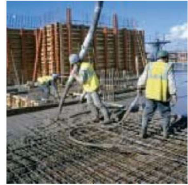
FIGURE 12–22 Steel rods around which concrete is poured for strength.
